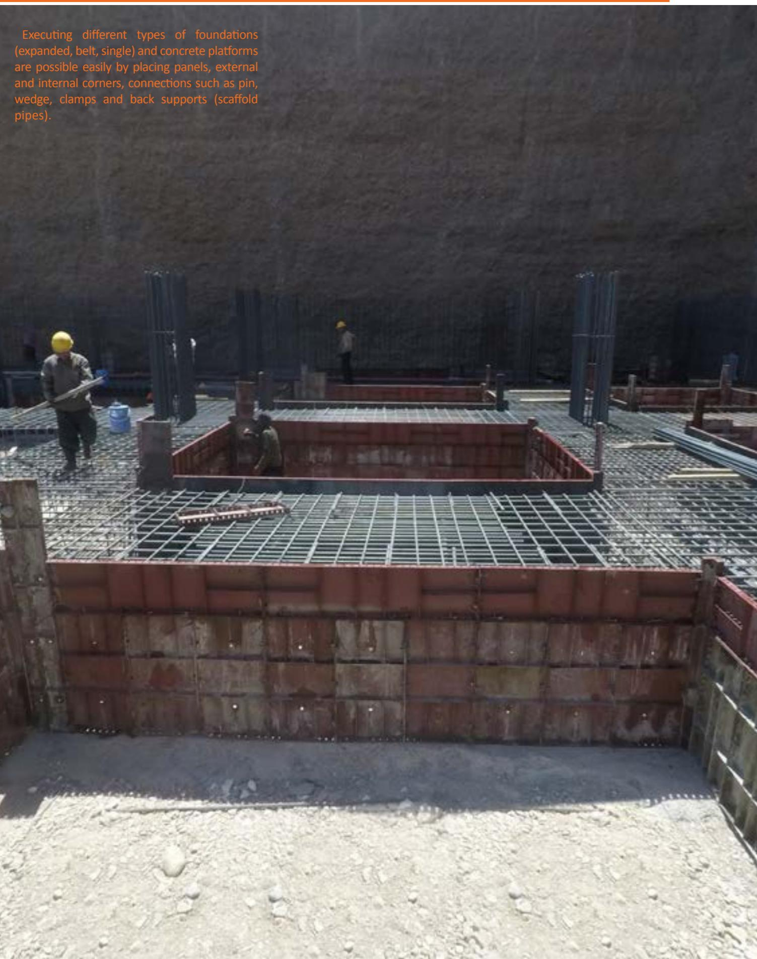
Executing different types of foundations (expanded, belt, single) and concrete platforms are possible easily by placing panels, external and internal corners, connections such as pin, wedge, clamps and back supports (scaffold pipes).
